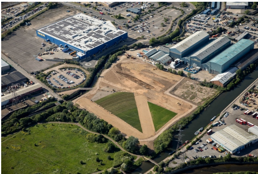
Aerial: Capping works
